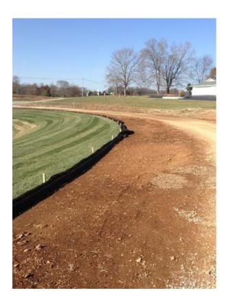
OVER 80% OF SEDIMENT AND POLLUTANTS ARE REMOVED AND RETAINED FROM WATER IN RECYCLED WOOD MATERIAL FILLER
