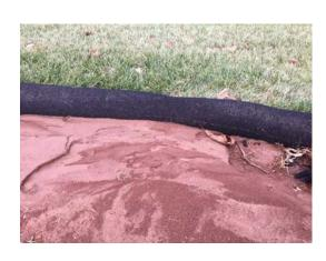
OUR SOCKS ALLOW WATER TO FILTER THROUGH THEM, SLOWING FLOW AND ALSO CAPTURING SILT AND SEDIMENTS.
